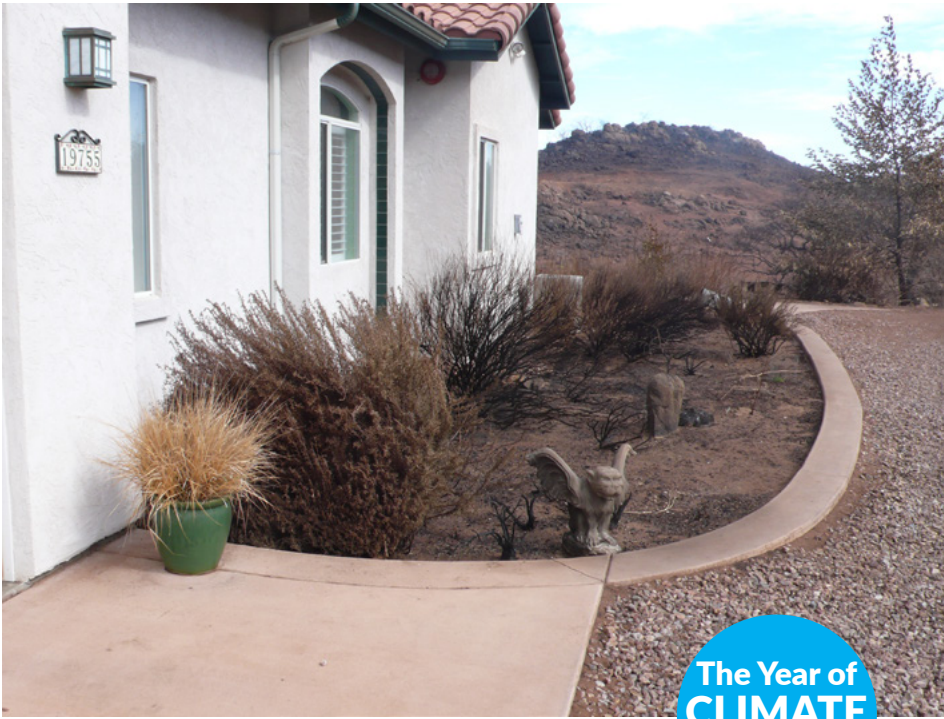
Left: Example of a home that survived the Witch Creek fire of 2007 with hydrated native vegetation planted in Zone 0. This may no longer be permitted under new legislation. Note there are no scorch marks on the white stucco. Below: Example of a home damaged by insufficiently irrigated junipers at its base.
