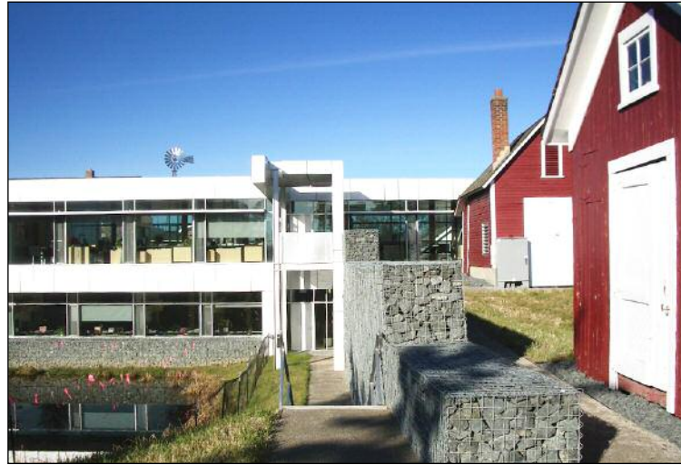
All buildings on site, including an historic farmhouse, were refurbished, relocated, and merged into the new campus design. To address grade changes, the site relies on many retaining walls formed with gabion baskets – wire baskets filled with recycled concrete, with only a veneer of crushed granite. Photo courtesy of Colin Brice, Brooklyn, New York.
