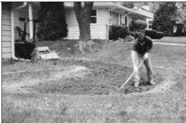
Note the roto-tiller in the background. To increase infiltration, it's easier to break up the soil and work in amendments with a tiller.
