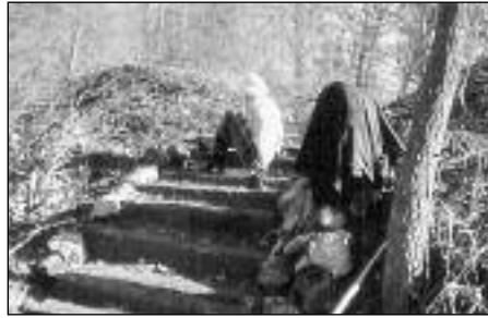
Student using her legs to leverage a rock into the border of the new access stairs.
